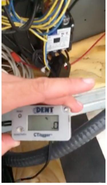
The logger is installed on the rooftop of the Ikea in Covina, CA. The logger is clamped around the hot lead on the compressor for the walk in freezer.
